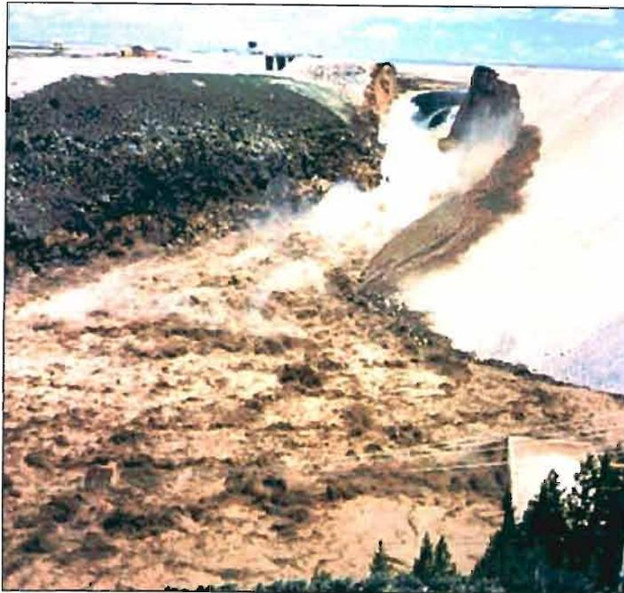
**Plate 2-5: The failure of Teton Dam as breach widens (Olson, 1976).**
