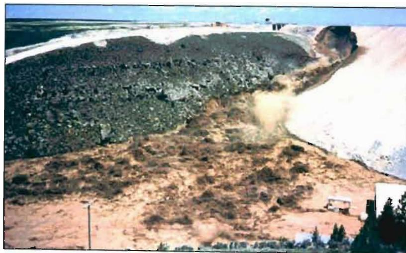
**Plate 2-4: Seepage reaches crest of Teton Dam (Olson, 1976).**
