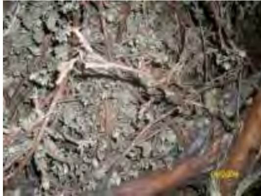
Figure 20: The interior view of a motebo roof
