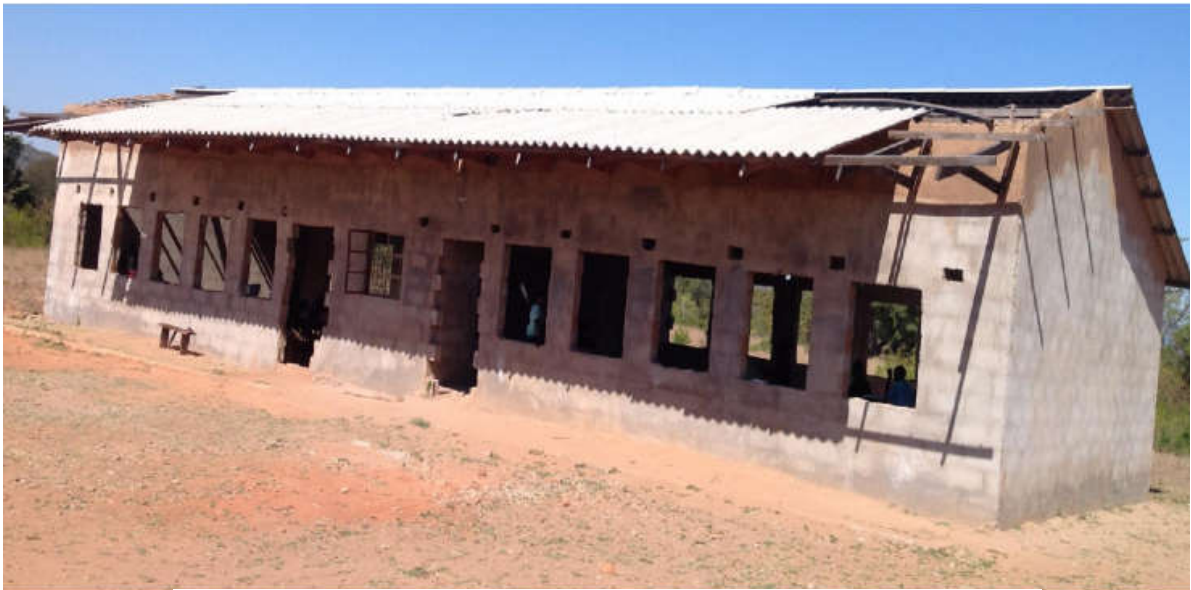
Plate 5.3 Pupils already learning in an uncompleted classroom at Sambo (Field data: 2015)
