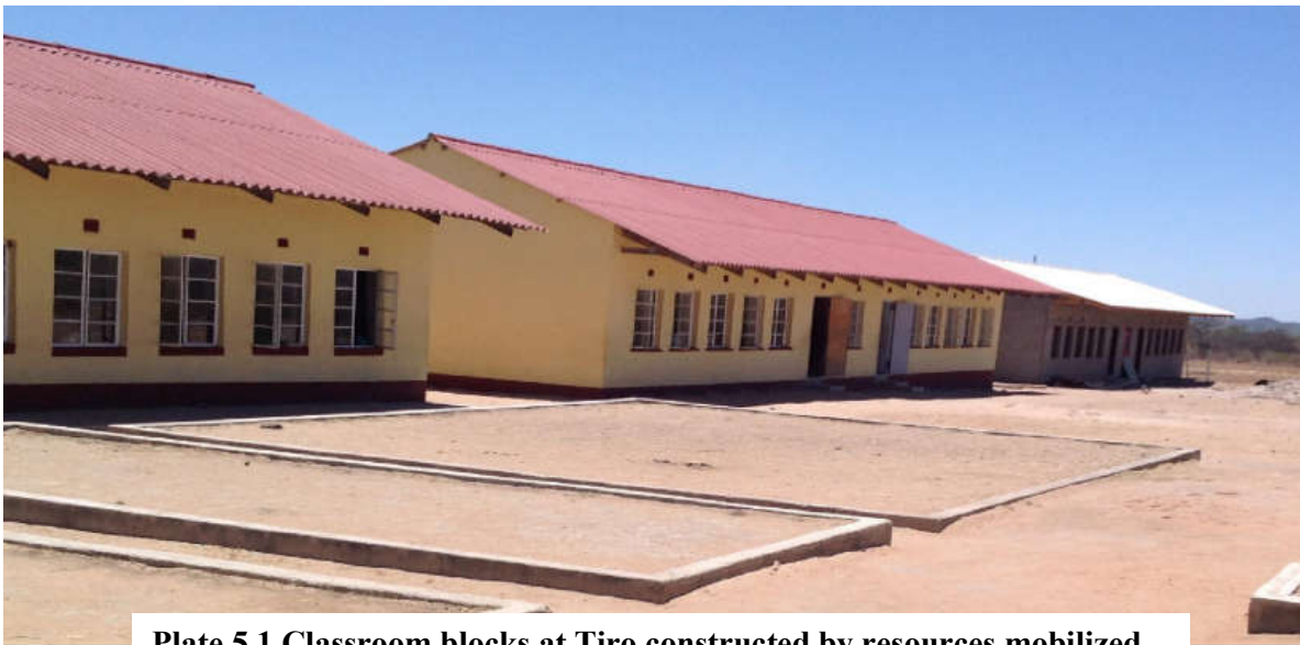
Plate 5.1 Classroom blocks at Tiro constructed by resources mobilized by land reform beneficiaries (Field data: 2015)
