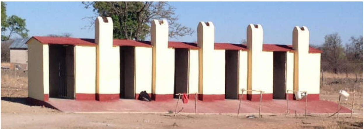
Plate 5.2 Toilets at Tiro constructed by resources mobilized by land reform beneficiaries (Field data: 2015)
