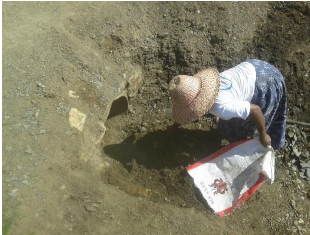
Figure 40: Parent working in the Zibambele road maintenance project: Site three
