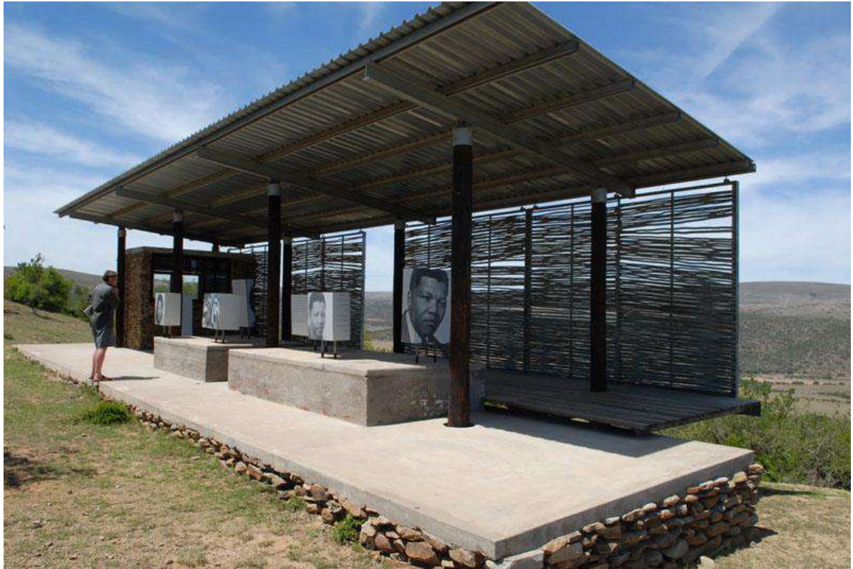
Plate 5.6 - Latte screens were used as shading devices and as a means of privacy and the screens were made from locally harvested wattle branches (Eicker, 2007; 18)
