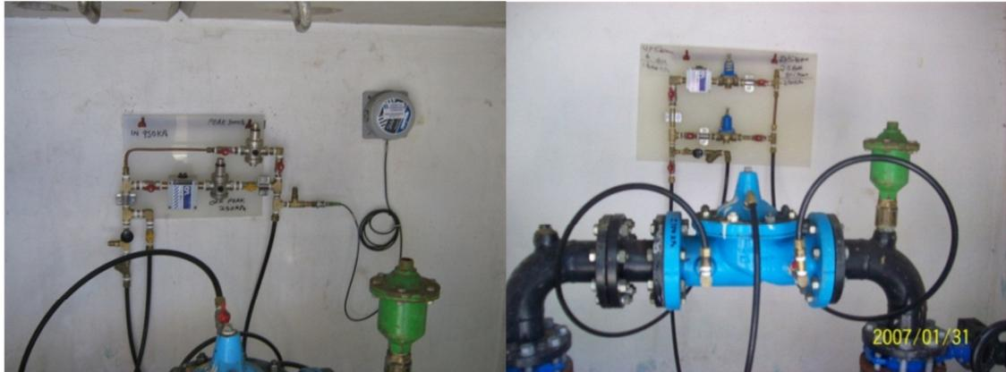
Figure 3.7: Dual pilot time control system connected to PRV
