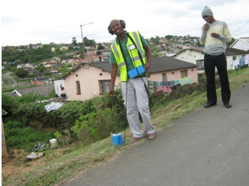
*Figure 3.21: Trunk Main Leak Detection with Amplified Listening Stick. (Photo courtesy of Mr Chris Otto, 2010)*
