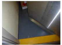
Fig. 5.3.17 Step threshold in solvents store door to prevent liquid from leaking out (By Author)
