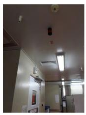
Fig. 5.1.18 Sealed ceiling and negative pressure monitors (By Author)
