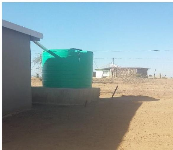
**Figure 7:** A Jojo tank mounted outside a home for the capturing of rainwater.
