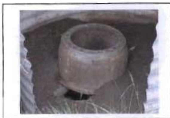
Plate 19: Surface water runoff penetrating pit latrine
